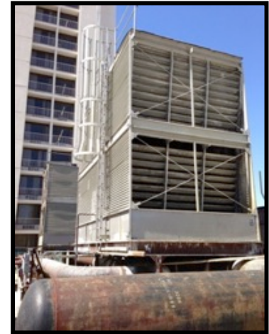
Cooling Tower Restoration
